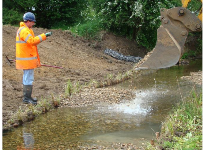
Banks graded and gravel introduced
