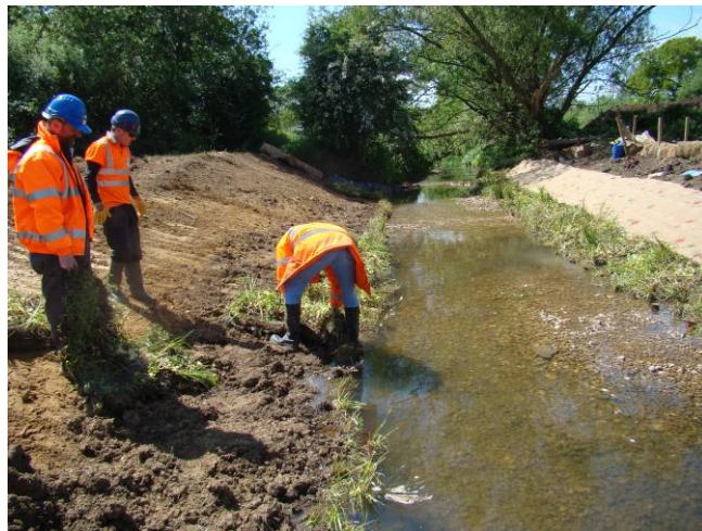
Installing pre-established coir pallets
