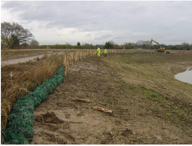
Rock Roll and Coir Roll Revetment Installation
