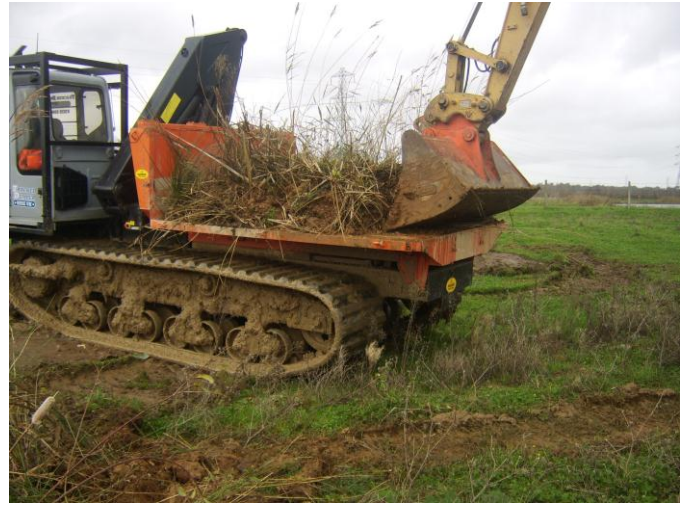
Existing reed habitat being translocated
