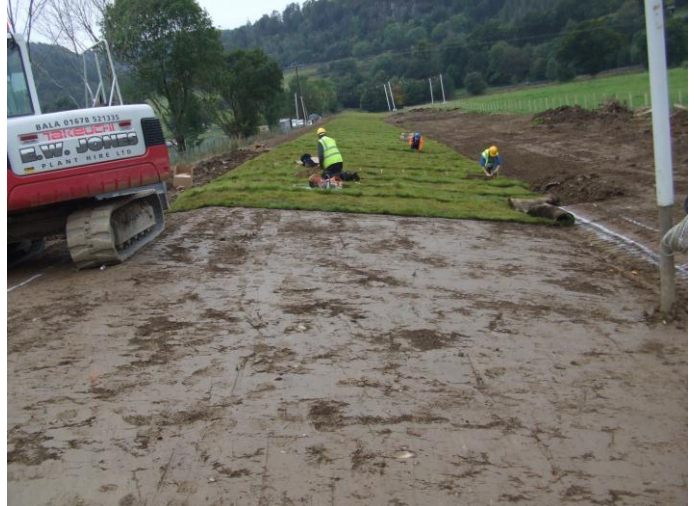
Installation onto well prepared surface
