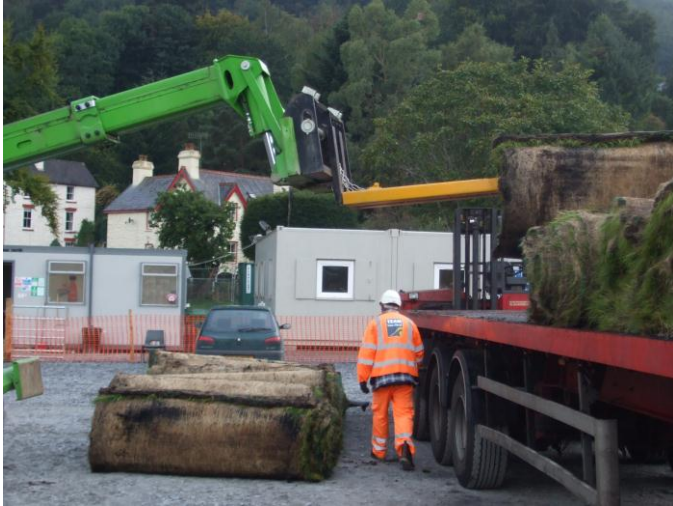
Shear stress turf delivered to site
