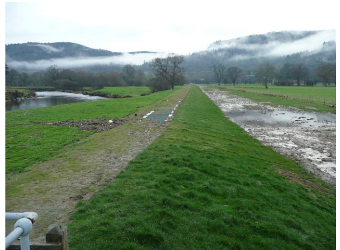
Aftermath of flood
